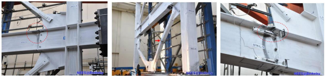
a) Local Buckling in top flange b) Brace Fracture c) Beam Fracture
