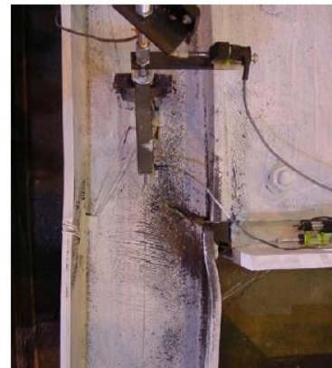
b) Fracture in column at 1.35% ODR
